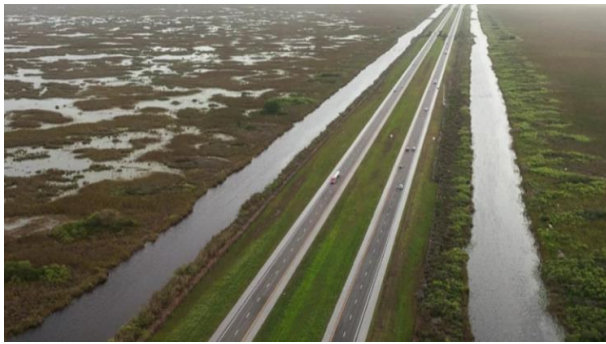
Fig. (1). Aerial view of long, straight, 4-lane divided highway with canals running parallel on both sides.
