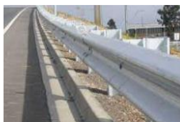
W beam barrier
