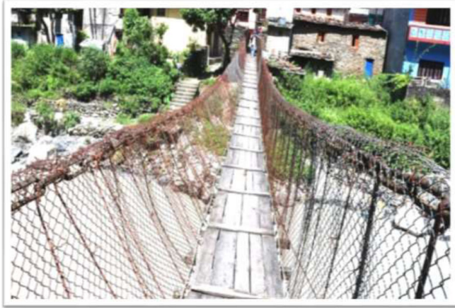
Fig. (4). Indigeneous baglung technology trail bridge over the myagdi khola, Myagdi.
