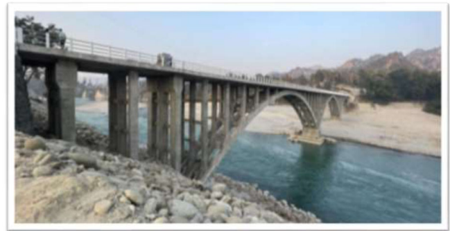
Fig. (12). Kochalighat kuine multi-span arch bridge over the karnali river.
