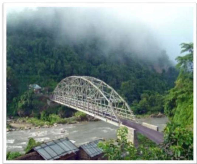
Fig. (14). Piluwa khola truss bridge.
