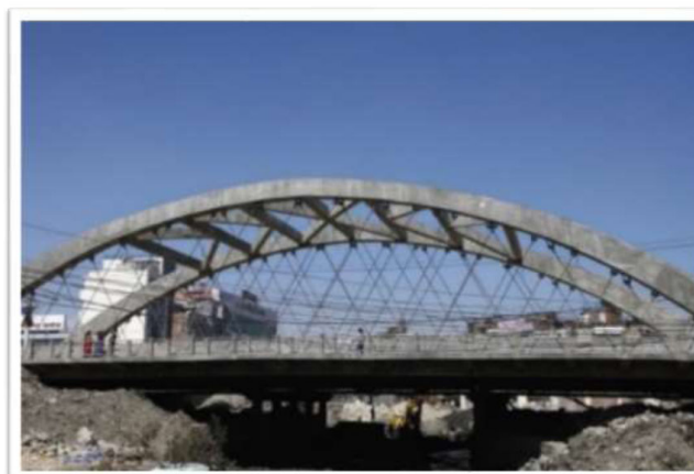
Fig. (7). Network arch bridge over the dhobikhola, Kathmandu.
