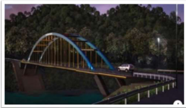
Fig. (9). Ramdi bridge over the kaligandaki river.
