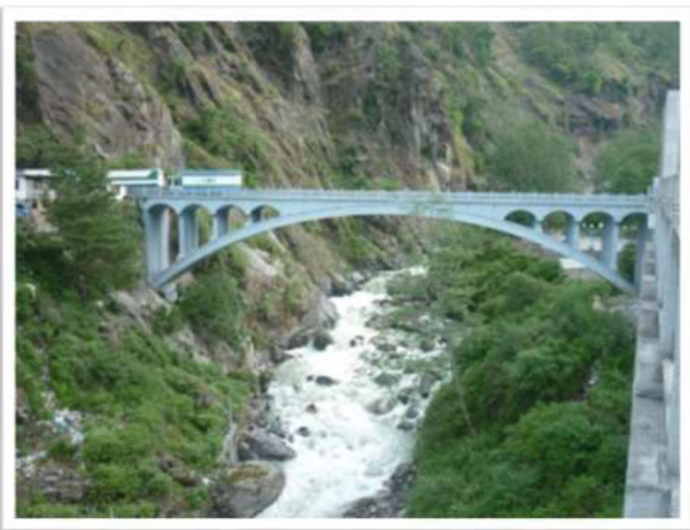
Fig. (10). Dech arch bridge over the bhotekoshi river in nepal-china border.
