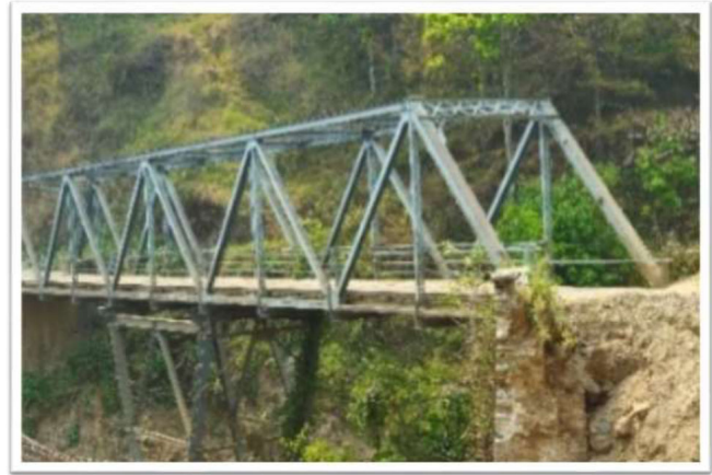
Fig. (3). Steel truss bridge over the tansin river.
