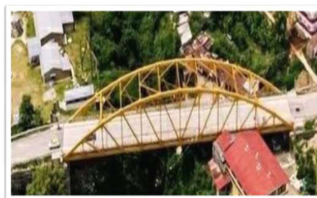
Fig. (8). Nadipur bridge over the seti nadi, Pokhara.
