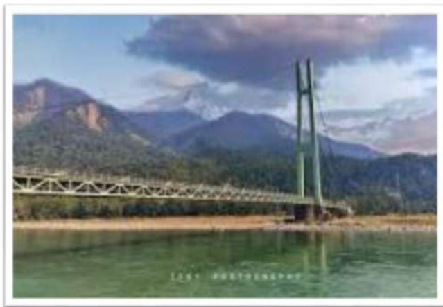
Fig. (17). Karnali cable-stayed bridge.
