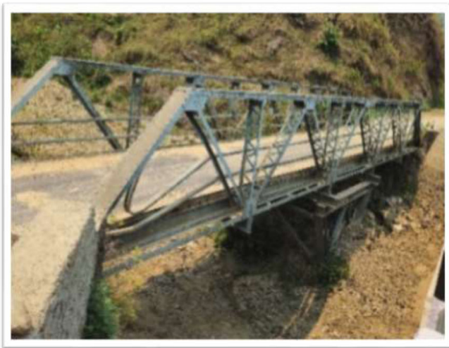
Fig. (2). Steel truss bridge over the nibuwater river.
