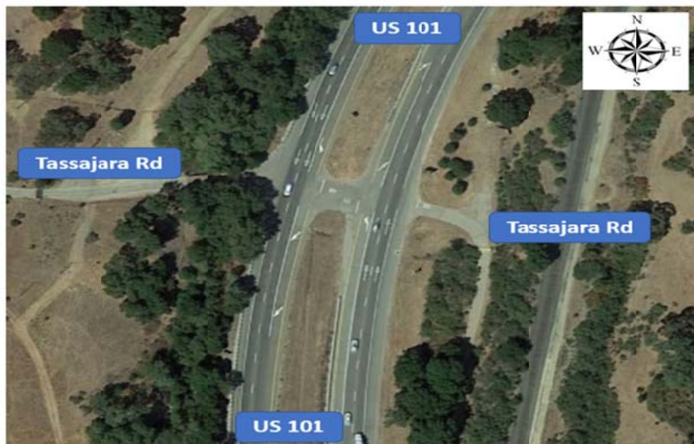
Fig. (2). The existing intersection on US 101 @ Tassajara Creek Road.
