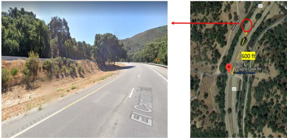
Fig. (3). The significant elevation difference between the two directions.
